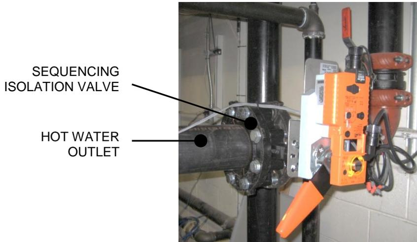
**Figure 2-13: Sequencing Isolation Valve Installed**
